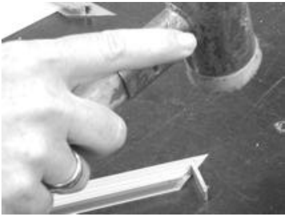
6. The hook profiles can be slightly hit on their ends for an easier assembly.
